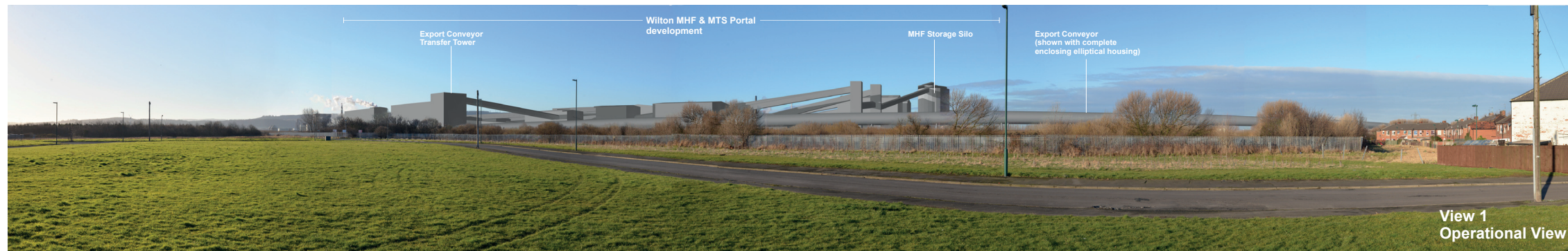
VIEW 1: Photographic illustration of Wilton MHF & MTS Portal development and export conveyor at stage 2 (complete structure)
