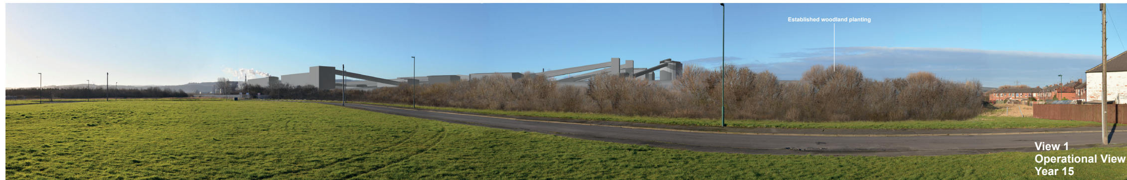
VIEW 1: Photographic illustration of Wilton MHF & MTS Portal development and export conveyor with foreground woodland planting established
