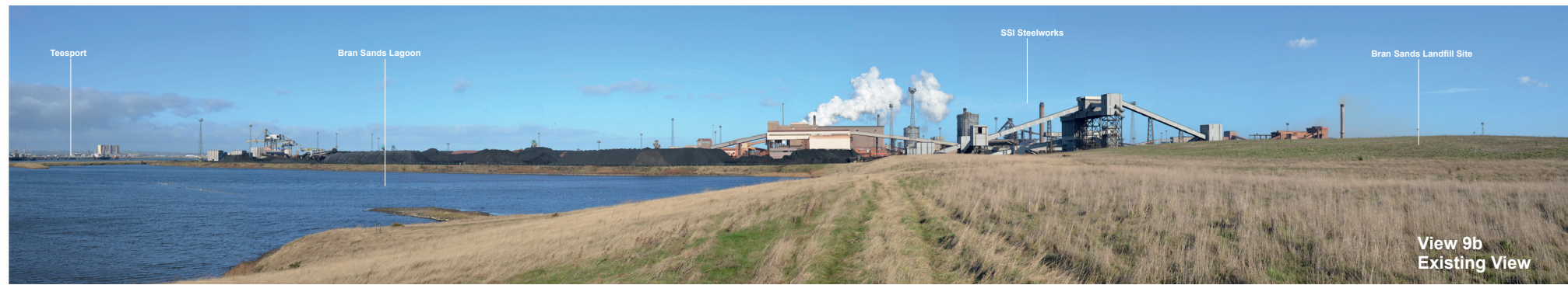
VIEW 9b: Existing view looking north from Bran Sands Landfill site towards SSI Steelworks site and Bran Sands Lagoon
