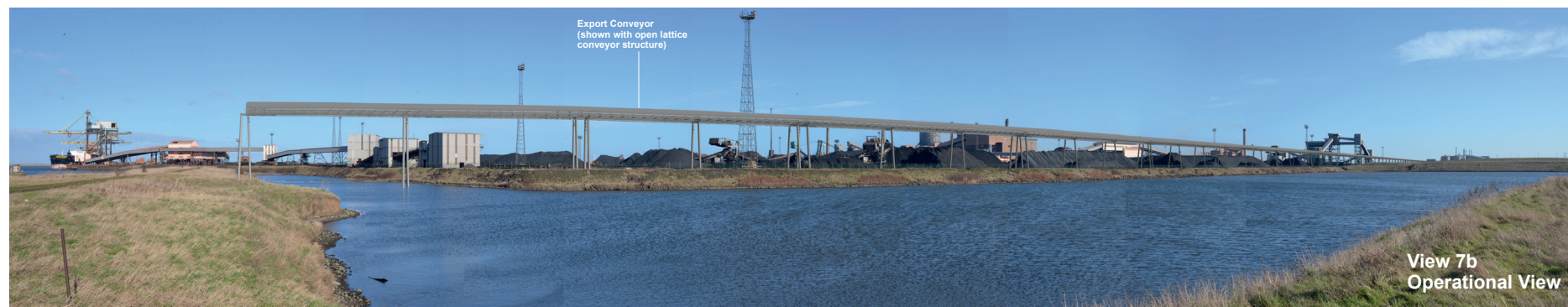
VIEW 7b: Photographic illustration of northern conveyor option at stage 2 (complete structure). Port facility and quayside structures not illustrated.
