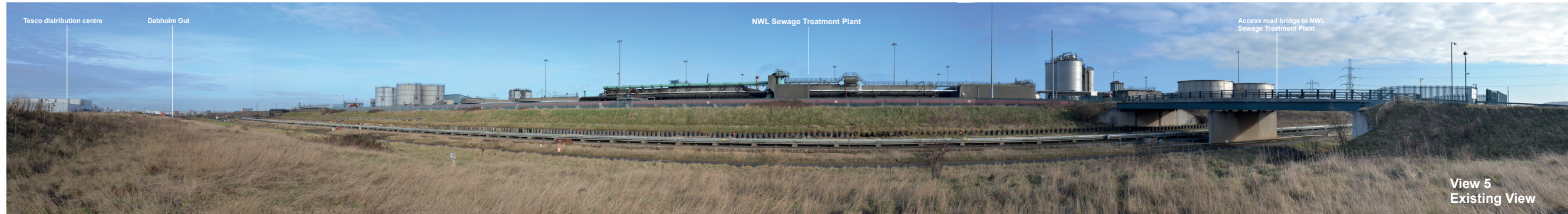
VIEW 5: Existing view looking north west from footpath 116/31/2
